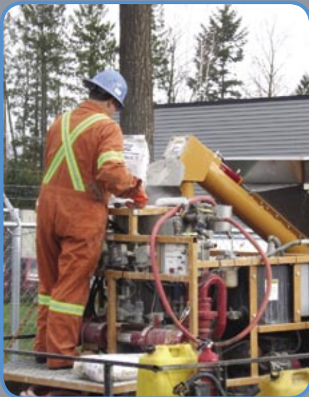
■ Grouting of bore hole.
