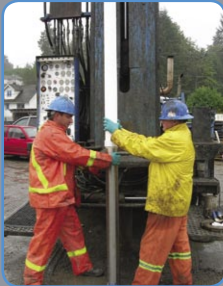
■ Installing stainless steel well screen with PVC riser pipe.
