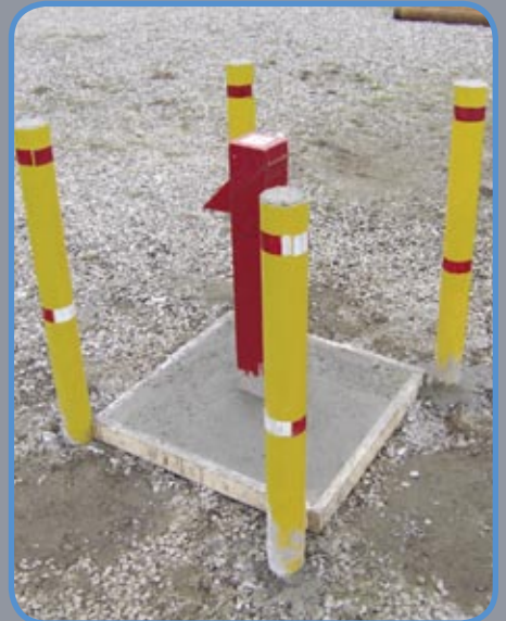
■ Finished observation well.
