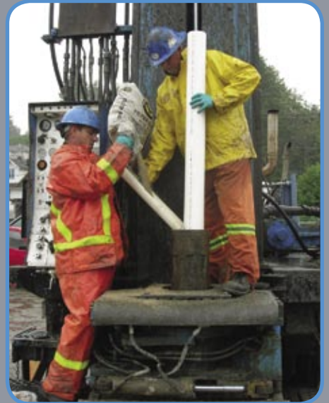
■ Pouring filter sand through temporary sonic outer steel casing.
