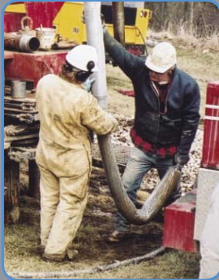
■ Extruding core sample using vibratory action.
