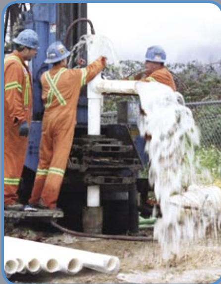
■ Well development in progress.
